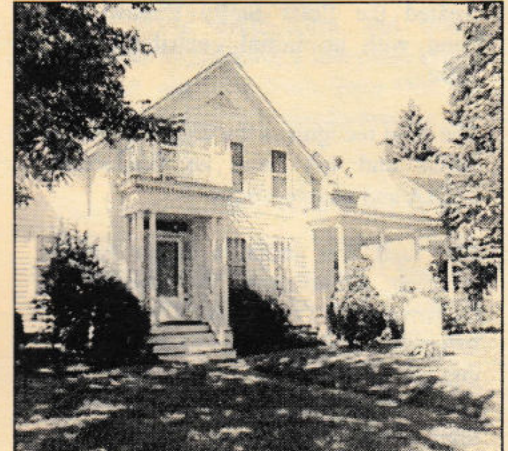
Saily House at 3 Cumberland Avenue
